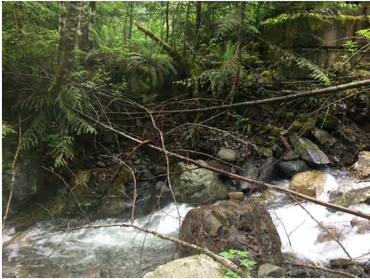
Downstream right bank riprap erosion
