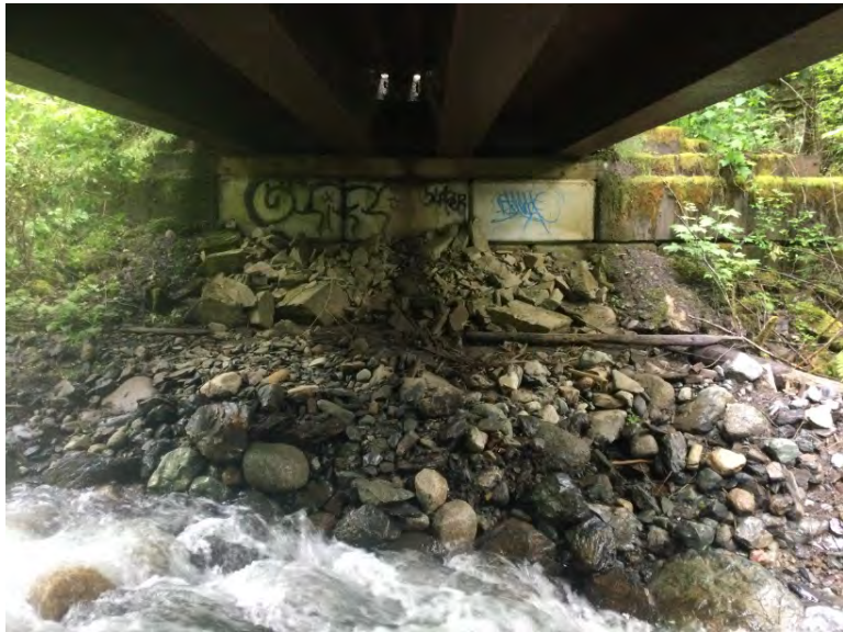
Left Bank Abutment when facing downstream
