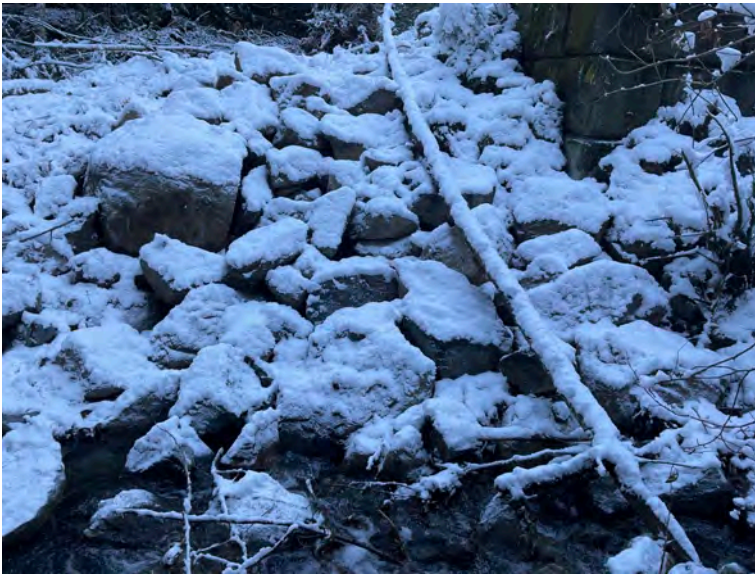
Downstream right bank riprap repair completed November 28, 2022
