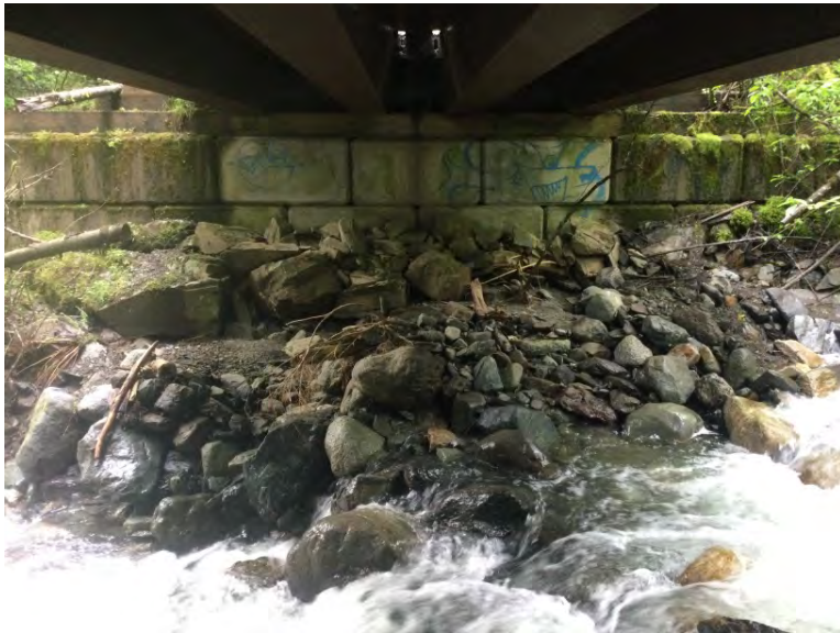
Right Bank Abutment when facing downstream
