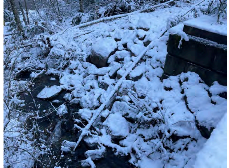
Downstream right bank riprap repair completed November 28, 2022
